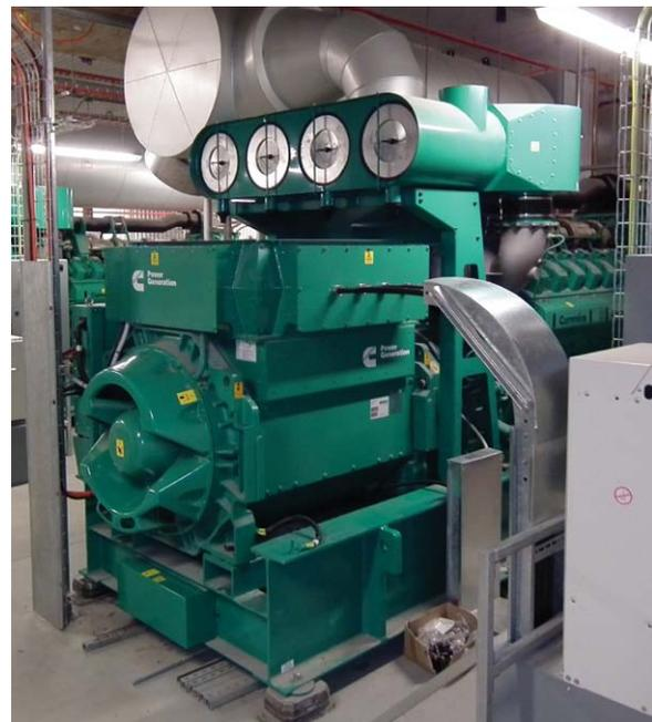
**Cummins installed a cogeneration plant at the flagship Royal North Shore Hospital in Sydney, Australia. The plant provides 4 MWe of base load power at peak periods, meeting the client's cost and efficiency requirements while producing less than 250mg/NM3 of oxides of nitrogen (NOx) emissions**
